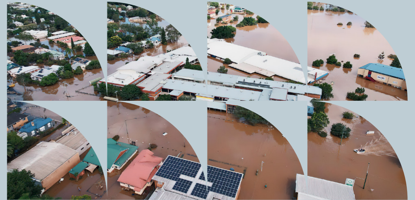
Above: Floodwaters inundated the Trinity Catholic College campus in Lismore in February 2022. Image: Trinity Catholic College.
